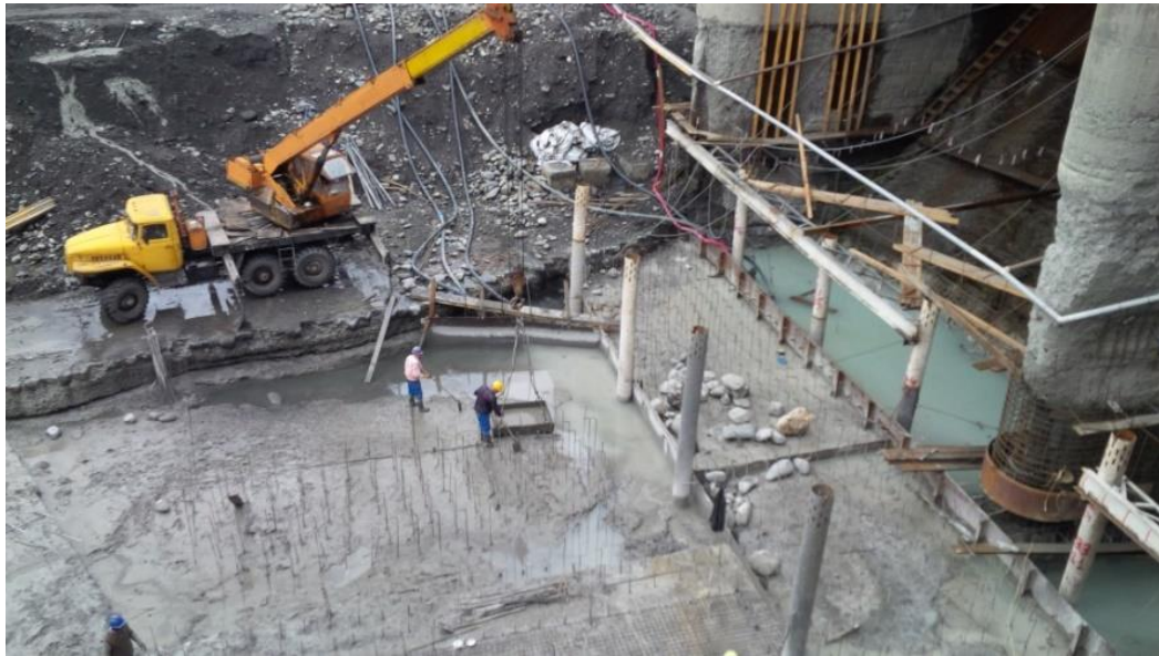
Photo 2 - The pit, concreted in the downstream side of the dam.
